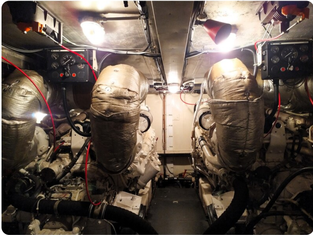
SANLORENZO SL 62 Engine Room
